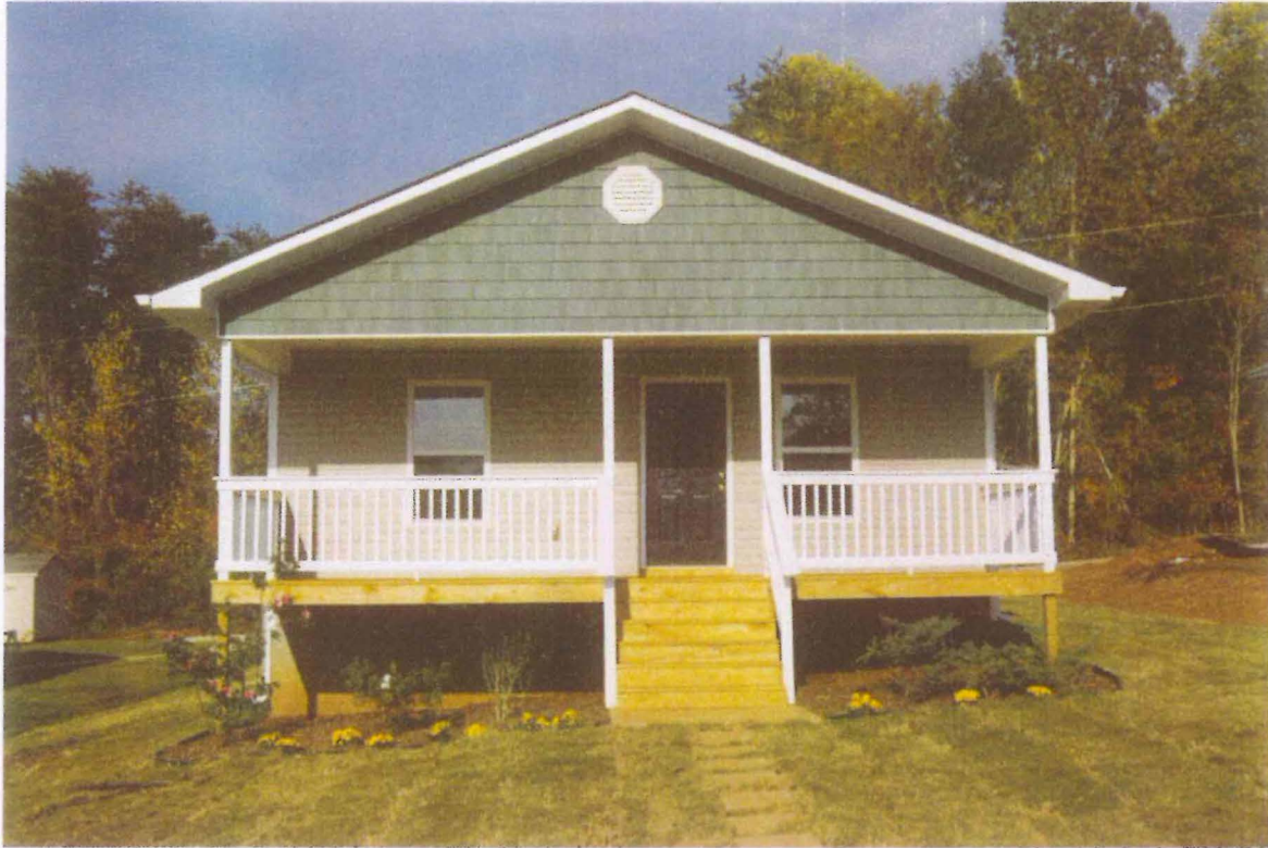
Example of pressure treated wooden porch posts, rails and steps
