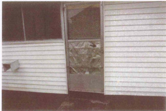
Back storm door: Replace with new half glass storm door
